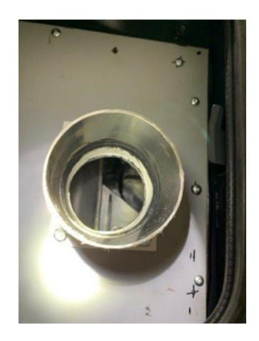
Drill 3" hole in filter housing cover in location of fresh air intake. Replace filter housing cover and seal around pipe.
