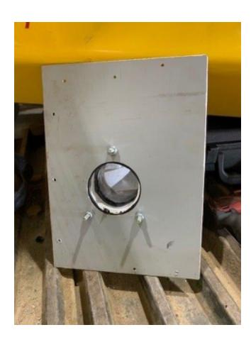
Seal perimeter of fresh air intake with silicone.
